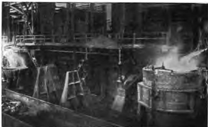
FIG. 196.—Drawing Steel from Open-Hearth Furnaces.
